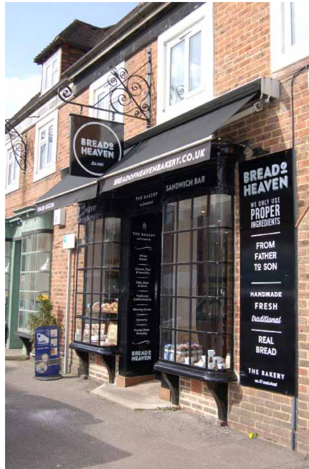
Figure 12. West Street, Haslemere: The incorporation of a retractable awning on this shopfront does not dominate over the overall frontage and allows for flexibility of use. The awning blends into the shopfront in terms of colour and is of a traditional style that complements and enhances the shopfront.
